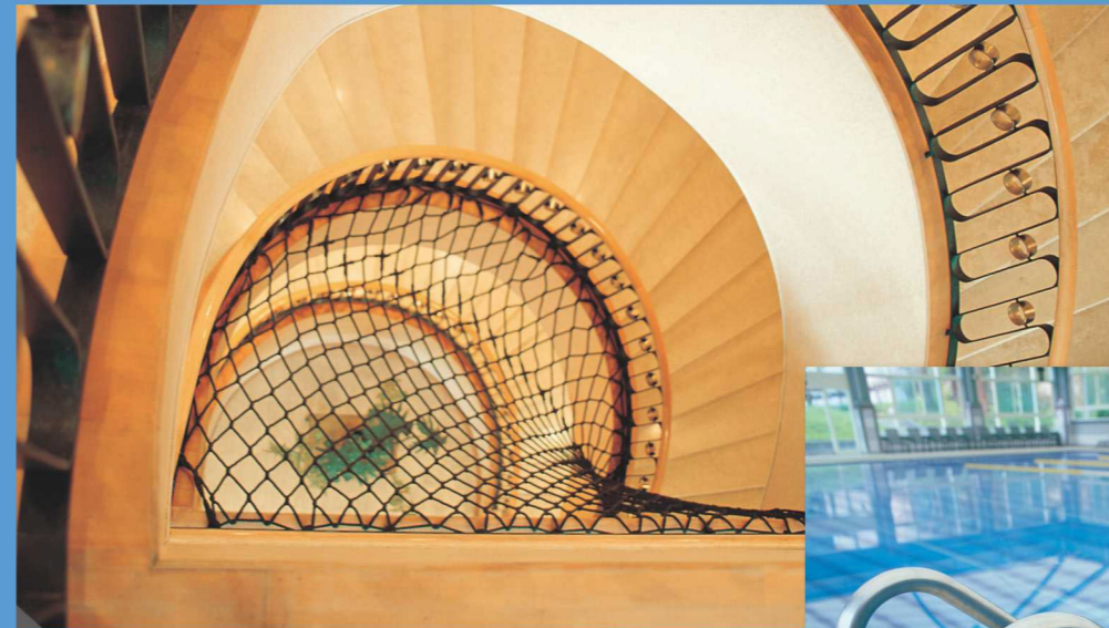
樓梯間安全網 Staircase Safety Net
